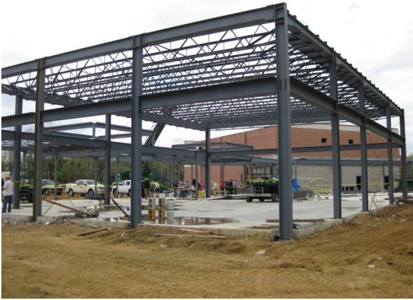
Banquet Facility - Concrete slab and structural steel finished
