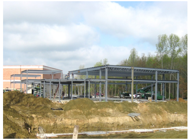
Banquet Facility - Concrete slab and structural steel finished
